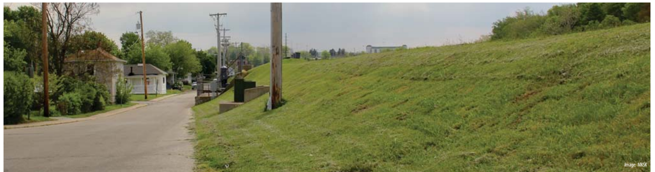
PUMP STATION ACROSS FROM RACE STREET
