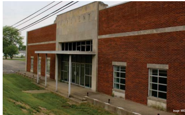
EXISTING AEROVENT CONDITIONS
