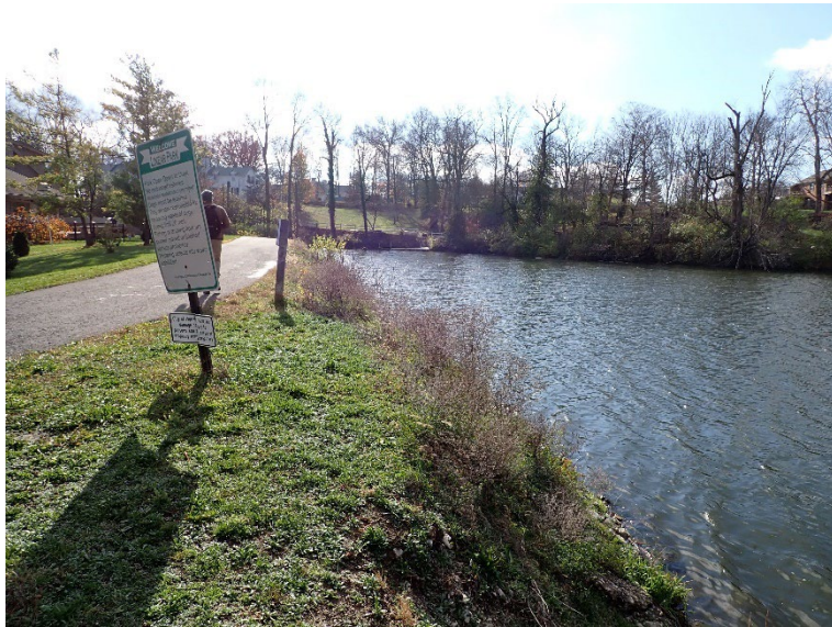
13. View of the upstream slope. Note the brush along the slope.
