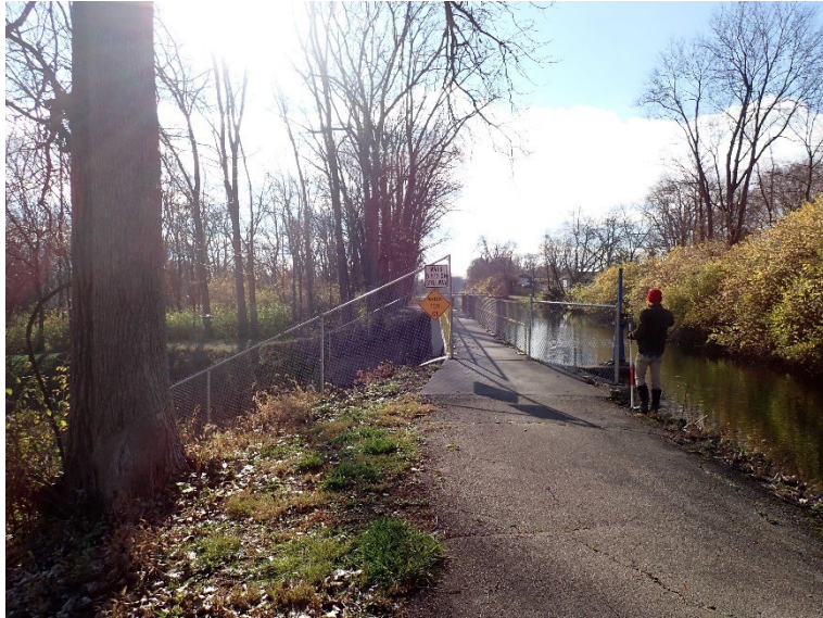
1. Canal path leading from Swift Run Lake Dam to principal spillway #1.
