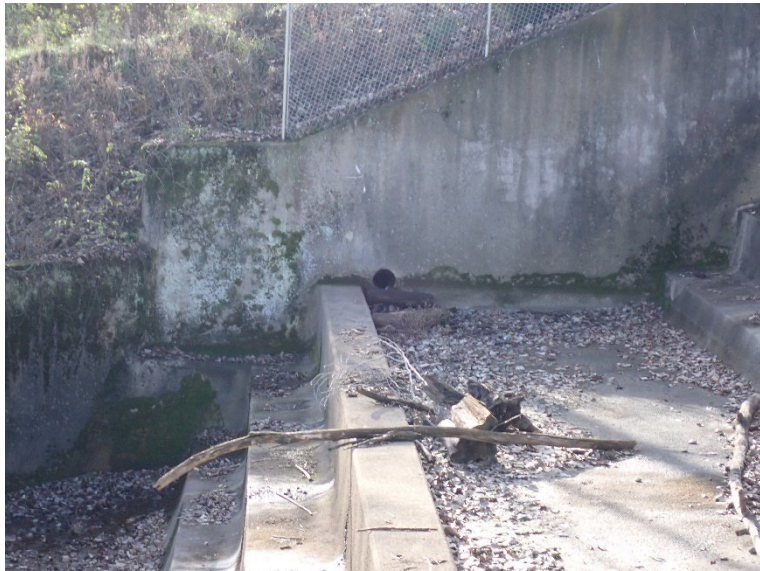
4. Closer view of the pipe opening in the right sidewall.
