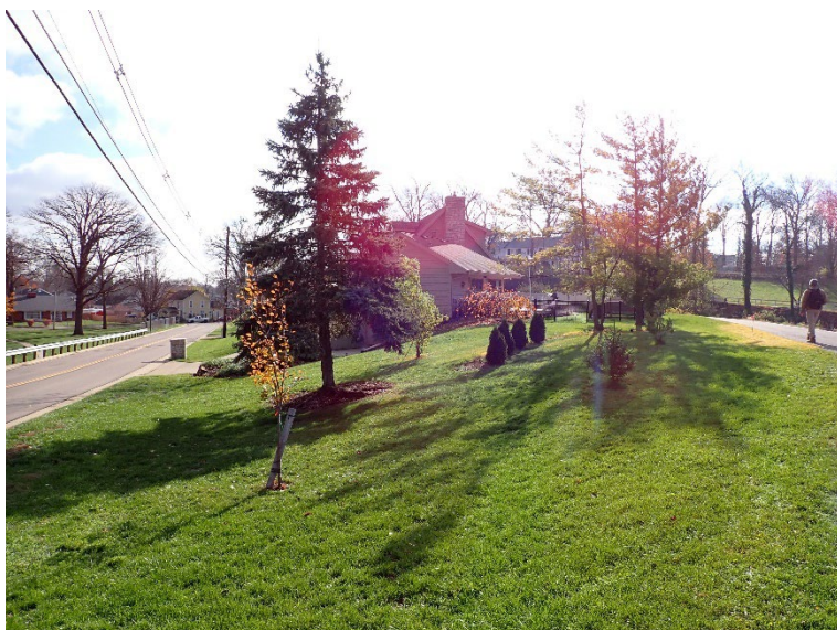
15. There is a house, a swimming pool, and landscaping trees and bushes in the downstream slope.
